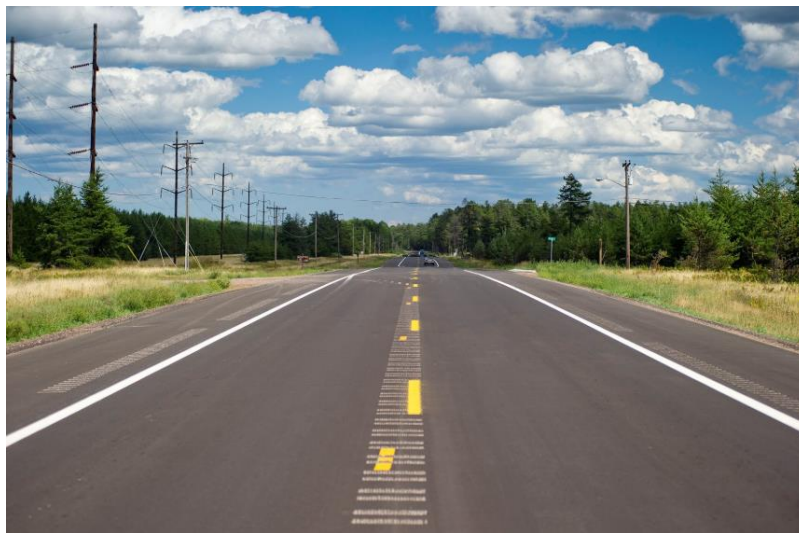
Figure 35. Centerline and Shoulder Rumble Strips.
